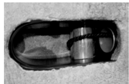
Guide box cast in concrete
