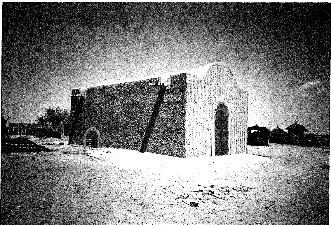
Photo 10: Cereal bank, Niger; low openings for ventilation and maximum useable space
