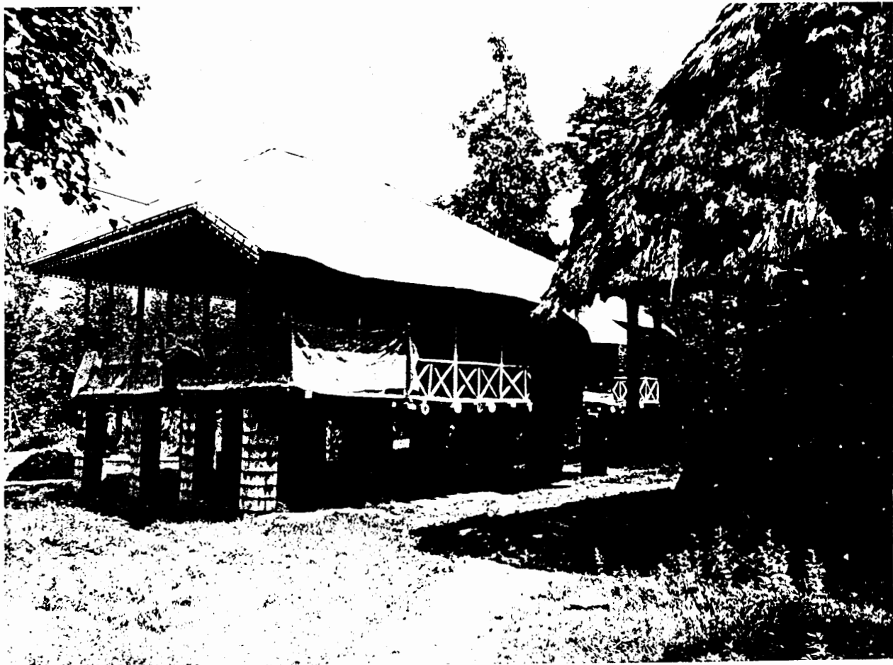
Concrete block columns have replaced wooden blocks used traditionally to raise the timber platform of the houses in order to avoid flood damage.
