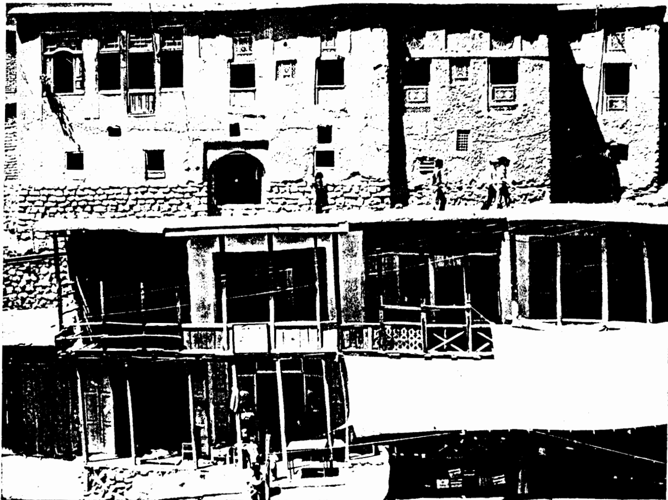
The upper level of the bazaar in Masouleh contains shops in a single row against the side of the mountain as in the same pattern as the housing.
