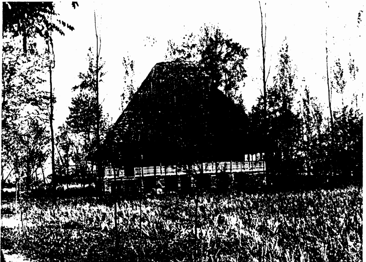
In the marshlands of the Sefidrud delta where flooding is likely, the houses are built on timber platforms that are raised from the ground on stilts.
