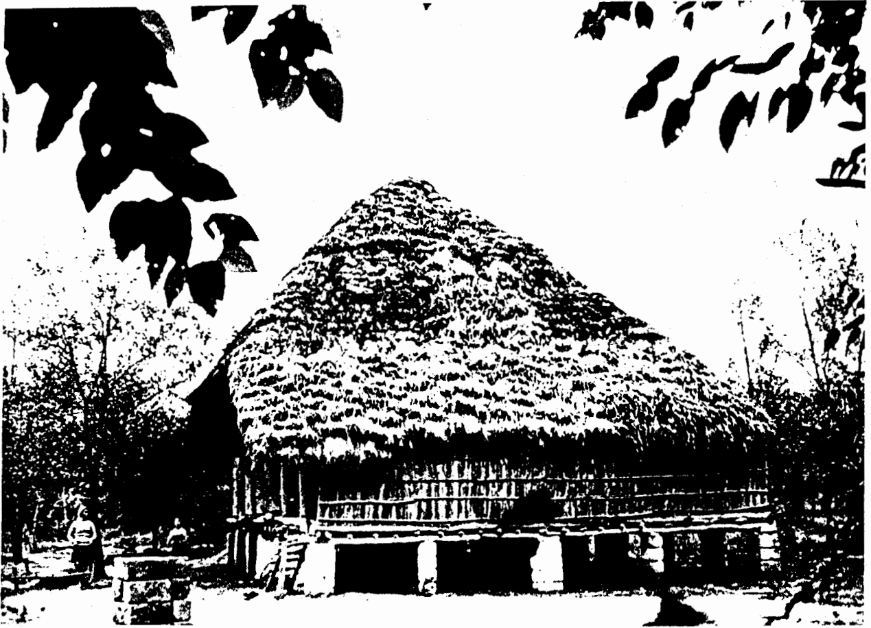
In the marshlands of the Sefidrud delta where flooding is likely, the houses are built on timber platforms that are raised from the ground on stilts.
