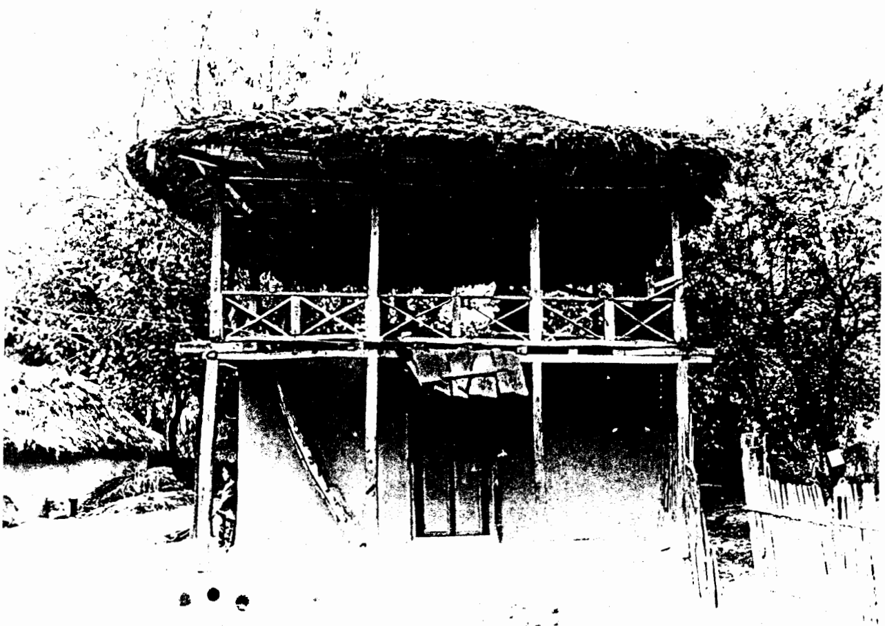
The nepari has an enclosed room on the ground floor and a shaded, well ventilated open platform on the upper level which is inhabited during warm summer months.
