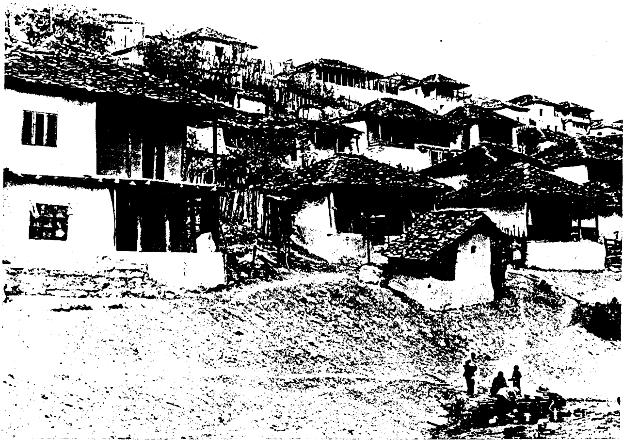
The village of Kodir, situated in a high mountain valley, exhibits a variety of house forms which are roofed by wooden shingles held down with stones.
