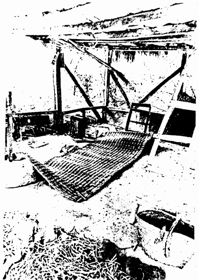
The nepari has an enclosed room on the ground floor and a shaded, well ventilated open platform on the upper level which is inhabited during warm summer months.
