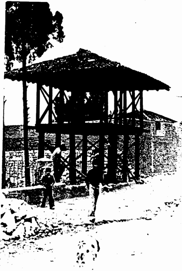
The nepari has an enclosed room on the ground floor and a shaded, well ventilated open platform on the upper level which is inhabited during warm summer months.
