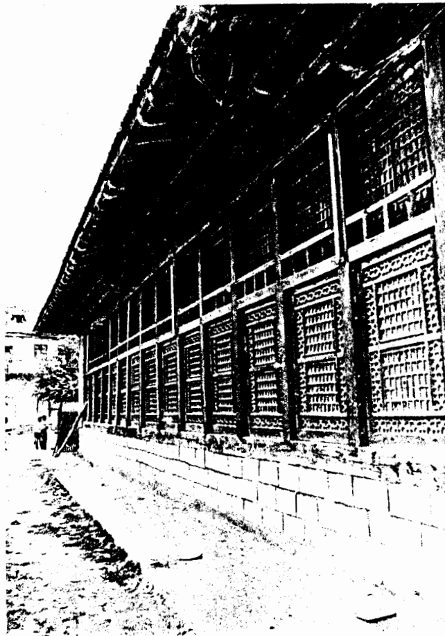
Timber framed buildings in Rostam Kola are in some cases enclosed by intricately carved timber lattice panels.
