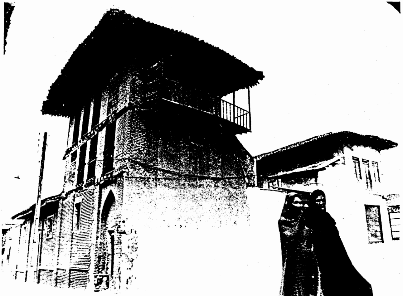
Buildings are two or three stories with brick walls and tile
