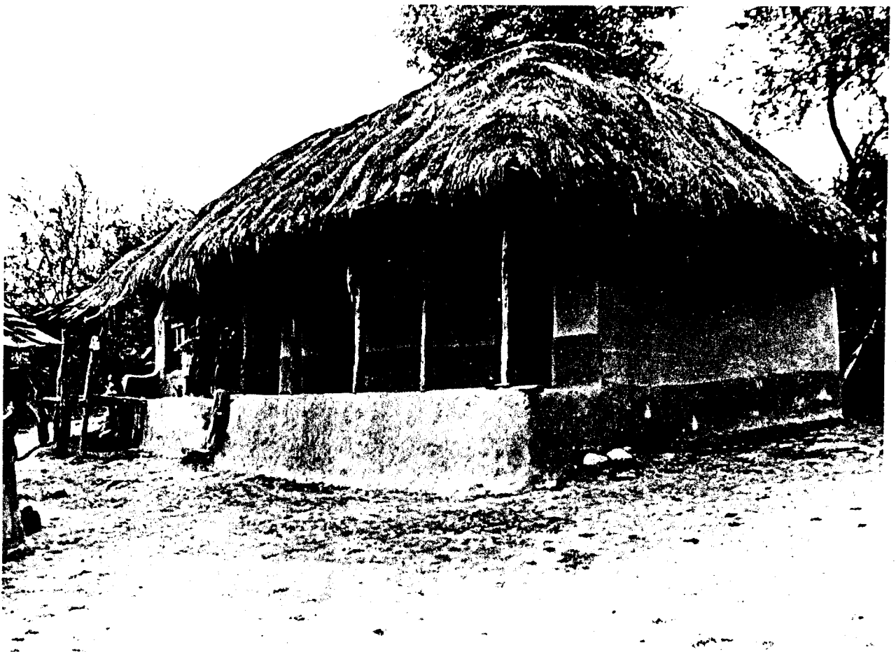
The basic house can be expanded horizontally to include two, three, or four rooms facing onto an aivan.
