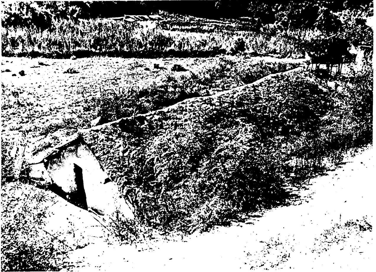
Mud roofs, normally flat, are built with a pitch in this village, west of Kojur.
