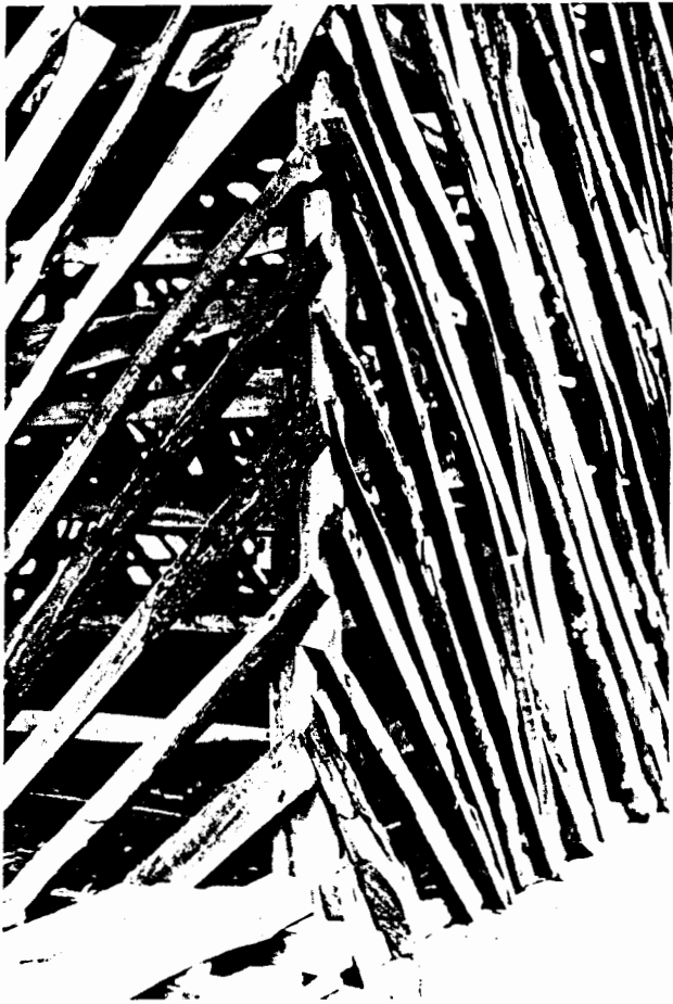
Walls made of timber lath and mud packing. These walls have either diagonal lathing (above) or horizontal lathing (below).
