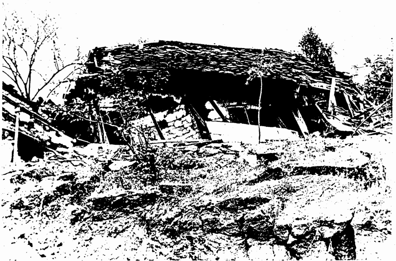
This house collapsed during a landslide. Diagonal bracing in the framing would have helped to resist collapse (Galand Rud).
