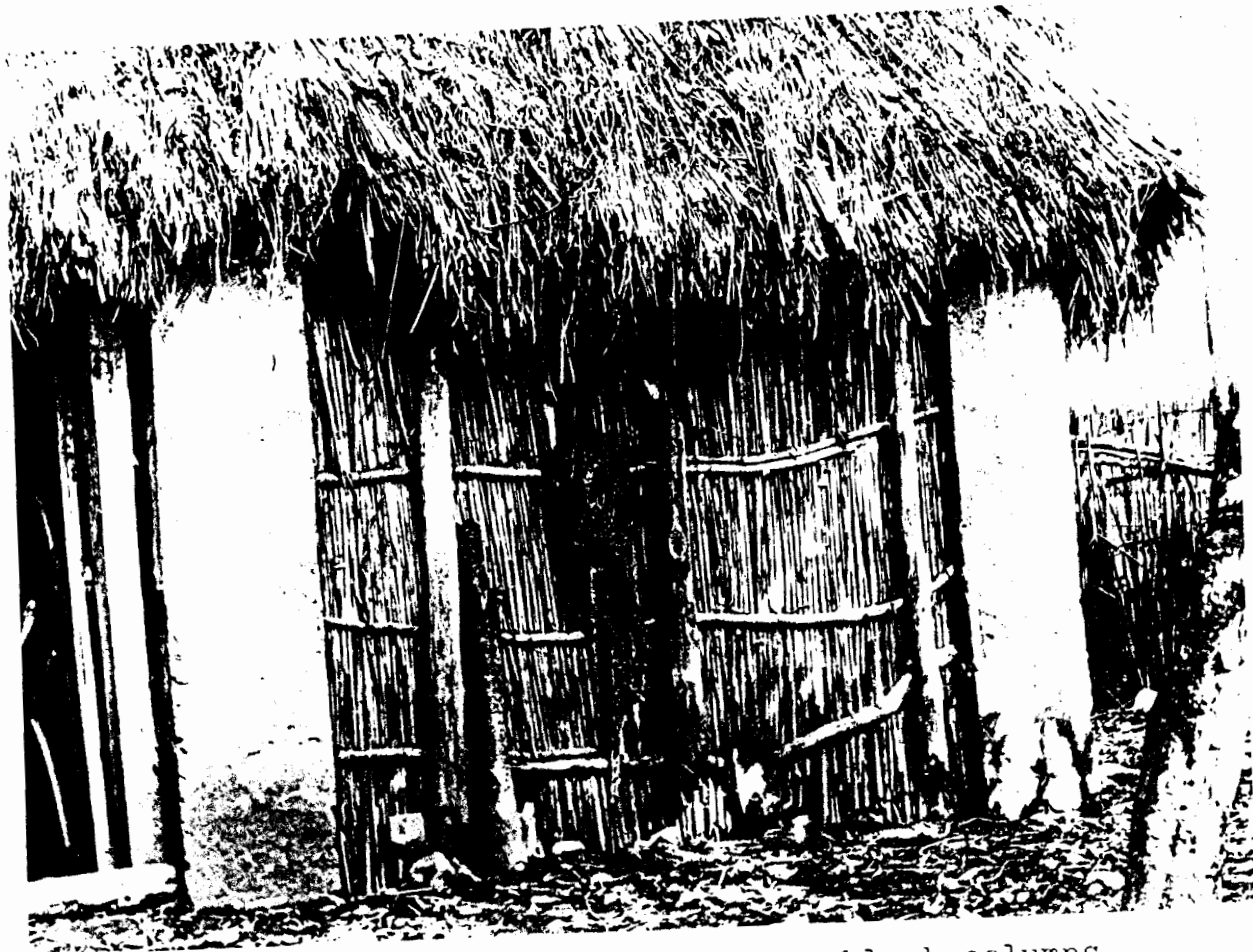
Reed wall supported between two concrete block columns (Shijan).
