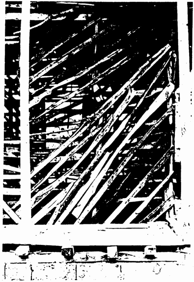
Walls made of timber lath and mud packing. These walls have either diagonal lathing (above) or horizontal lathing (below).
