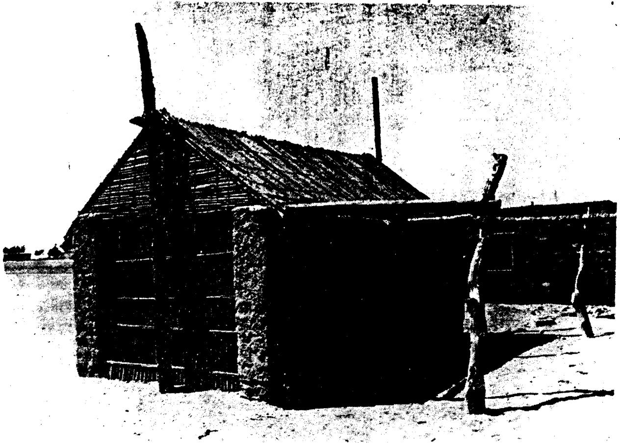
Mud Brick posts, supporting barasti screen walls.
