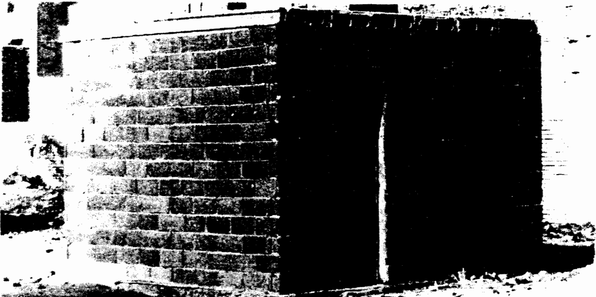
Reinforced concrete roofs are a solution, though very expensive.
