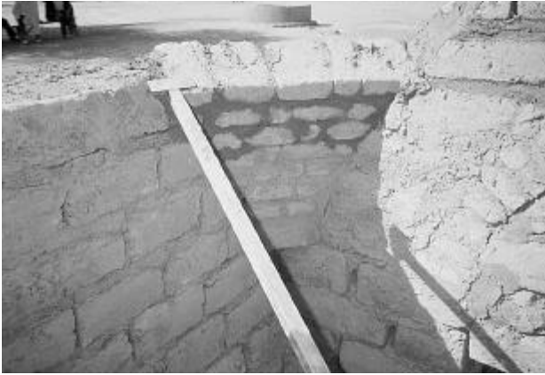
Fig. 11 The radial arm showing the placing of bricks in a pendentive, the lower part of the corner of a dome.
