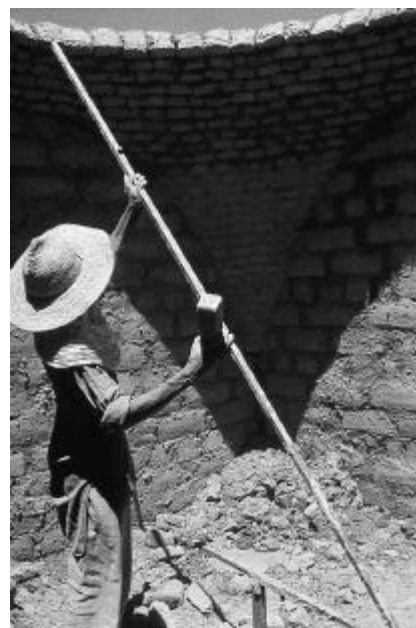
Fig. 8 Using the radial arm in dome building. The arm gives the placement and the angle of every brick.
