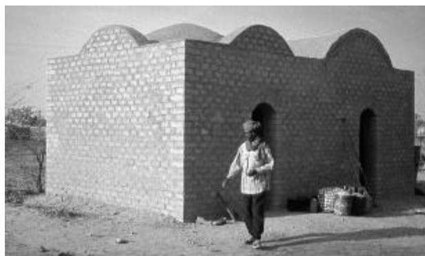
Fig. 12 A small two-roomed house, with one domed room and one vaulted room, provides a good training module.
