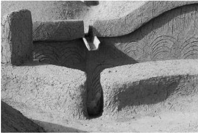
Fig. 10 Smooth curves and large gutters help ensure a good flow of water off the roof.
