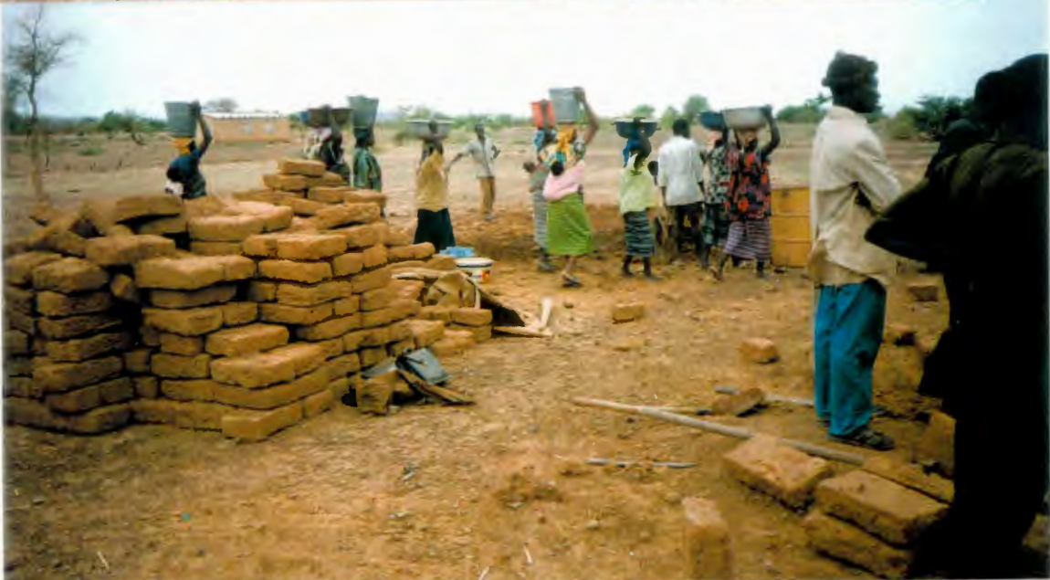
Photos 11 and 12: Village youth organisations in Burkina Faso undertake to provide the correct quantity of bricks, and on site earth, water and labour; only the skilled "woodless construction" building input is project-provided at this early "demonstration" stage.
