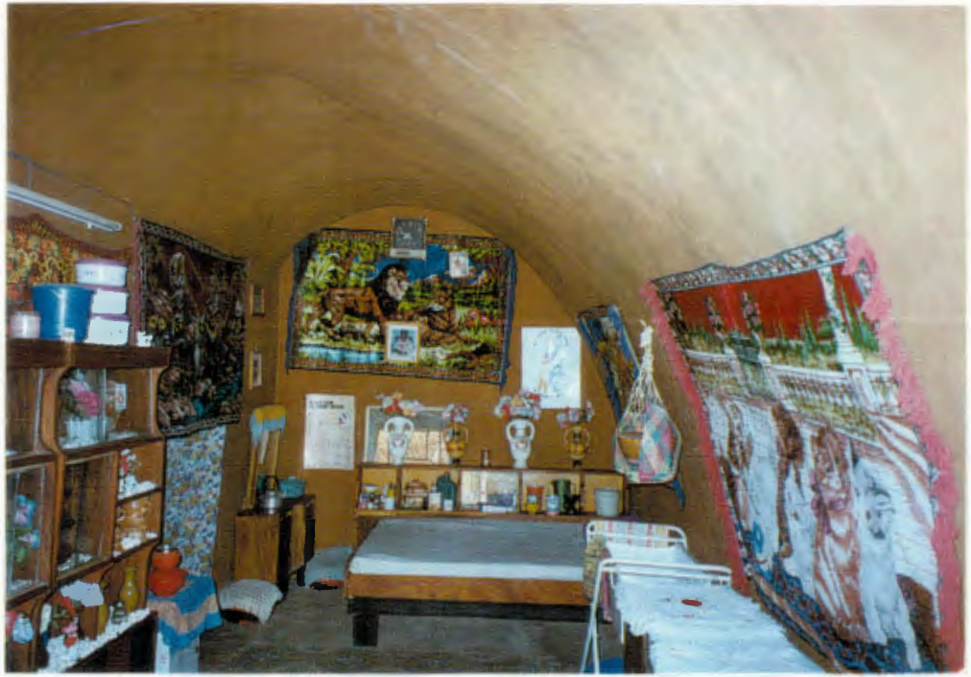
Photo 16: "Eccentric" vaults give more vertical wall space for modern needs, Mirriah, Niger.
