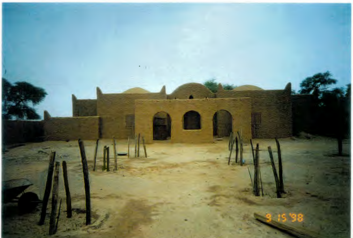
Photo 3: Recently completed (98) villa using a combination of vaulted and domed rooms, Iférouane.
