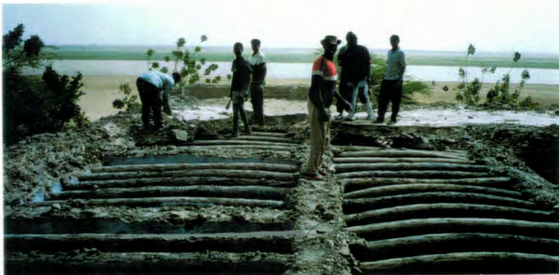
Photo 5: "Traditional" flat roof under construction showing massive use of timber beams.
