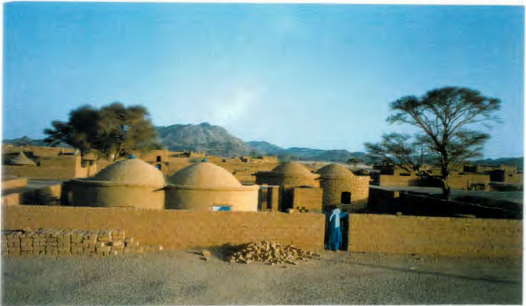
Photo 2: Combined domed rooms, built by an Iférouane mason for his own family.
