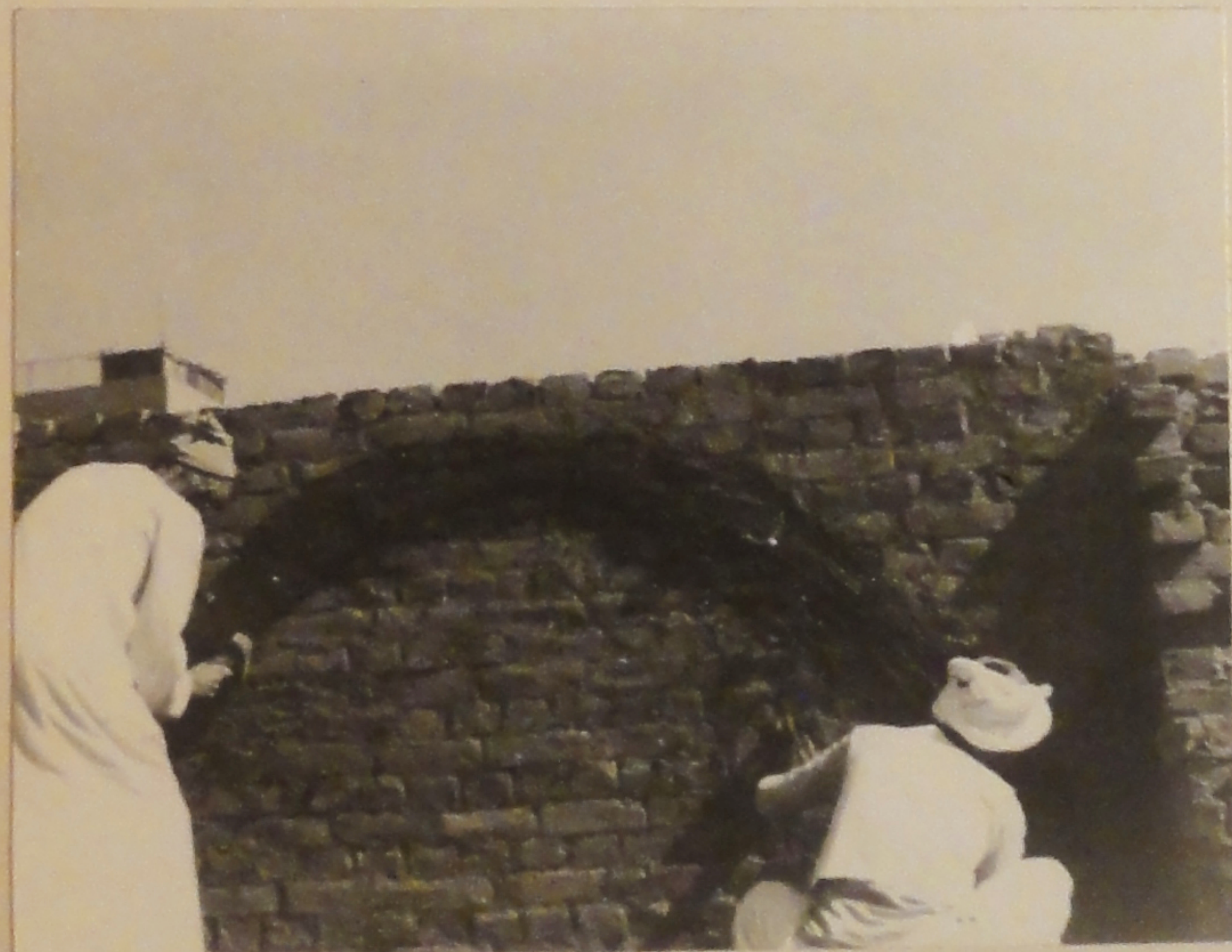
11 THE CURVE OF THE VAULT FOLLOWS A PARABOLA, THE MASONS ROUGHLY OUTLINE THE PARABOLA FREEHAND AGAINST THE END WALL. THEN WITH THE ADZE THEY TRIM THE MUD PLASTER TO GIVE IT A SHARPER OUTLINE.
