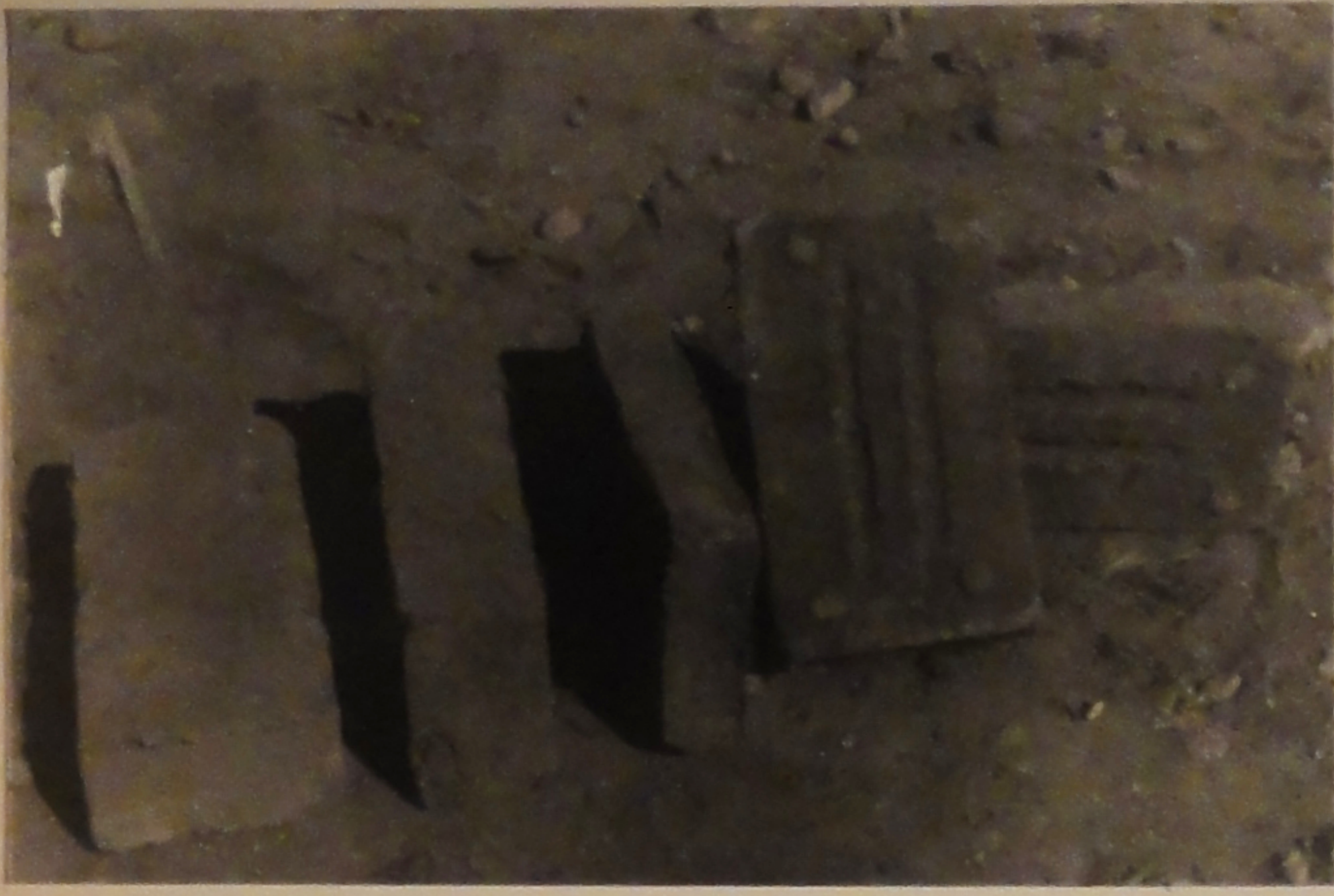
9 VAULT BRICKS ARE THINNER THAN STANDARD BRICKS, AND MADE WITH MORE STRAW THAN USUAL, FOR LIGHTNESS (120 LBS OF STRAW FOR ONE CUBIC METRE OF EARTH) MEASURING 25CM X 150CM X 5CM AND MARKED WITH TWO DIAGONAL GROOVES DRAWN WITH THE FINGERS FROM CORNER TO CORNER OF THE LARGEST FACE. THE GROOVES ENABLE THE BRICKS TO STICK TO THE MUD PLASTER BY SUCTION.
