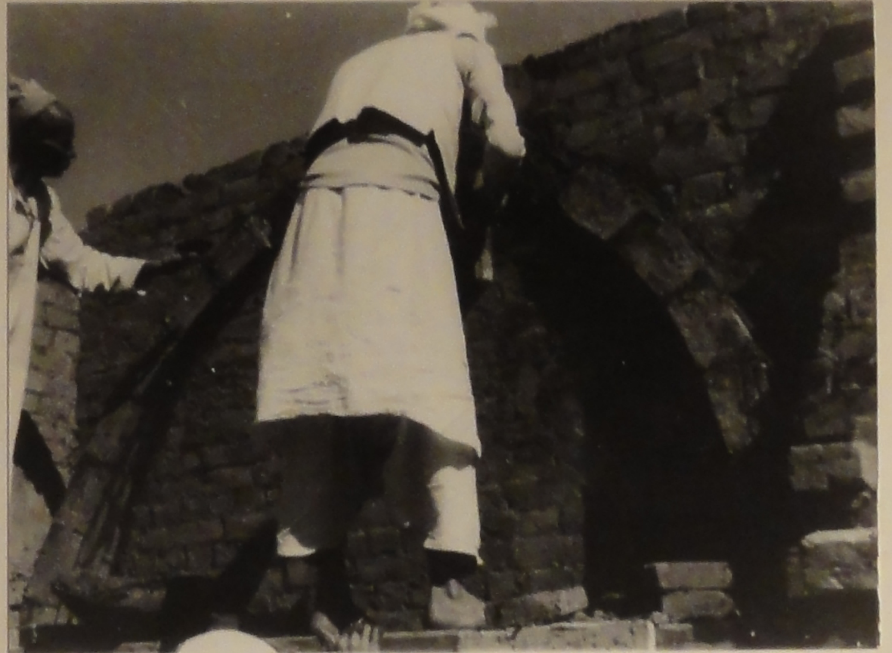
16 & 17 THESE TWO PHOTOGRAPHS SHOW THE TWO MASONS GRADUALLY BUILDING THE INCLINED COURSES OUT, EACH ONE RISING A LITTLE HIGHER ROUND THE OUTLINE OF THE PARABOLA, TILL THE TWO CURVED LINES OF BRICK MEET AT THE TOP.
