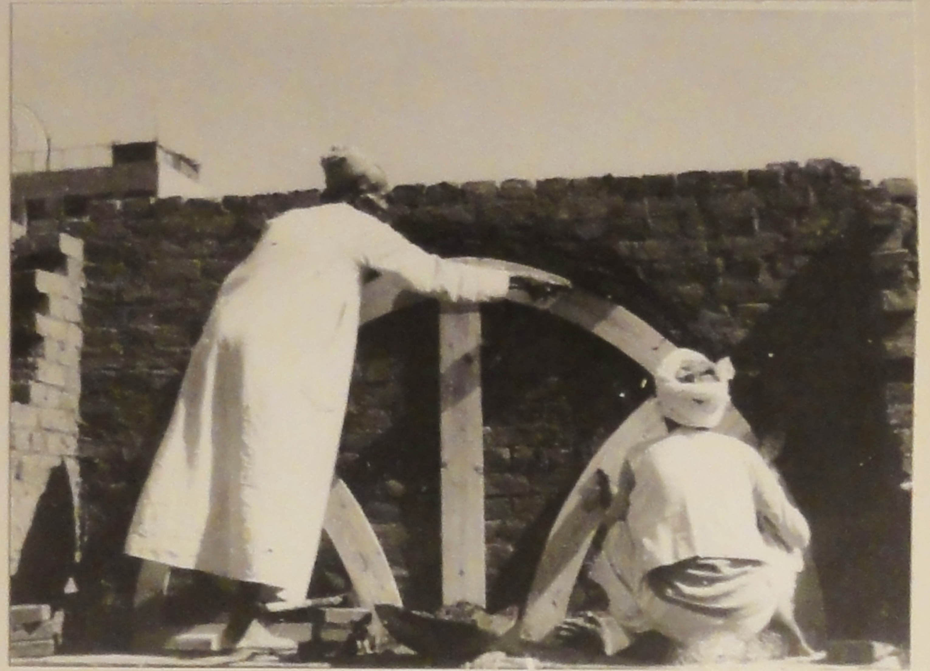
12 WHEN THE CURVE IS CORRECT AND SYMMETRICAL AND THE EDGES ARE CLEANED OFF WITH THE ADZE, A TEMPLATE CAN BE USED TO CORRECT THE CURVE AND TO CHECK THE WORK OF THE MASONS. THE PHOTOGRAPH SHOWS THE TWO MASONS CHECKING THE PARABOLIC CURVE WHICH THEY HAVE DRAWN FREEHAND AND THE TEMPLATE DESIGNED BY THE ENGINEER. THE TWO CURVES ARE ALMOST THE SAME.
