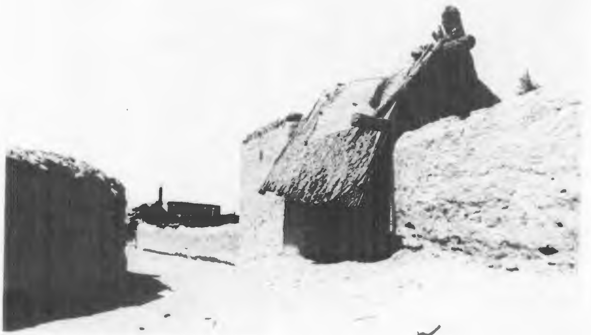
Fig 3.19 Winter Village Falaj al Qabael Note mud brick houses and added matting on berastî roof.
