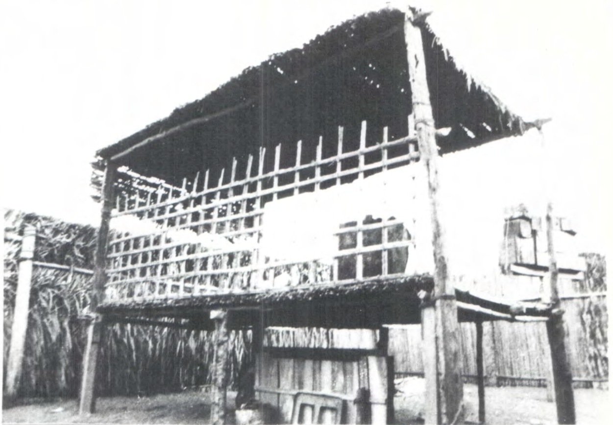
Raised platforms are often used for storing food. The introduction of insect and rodent guards would be an improvement.
