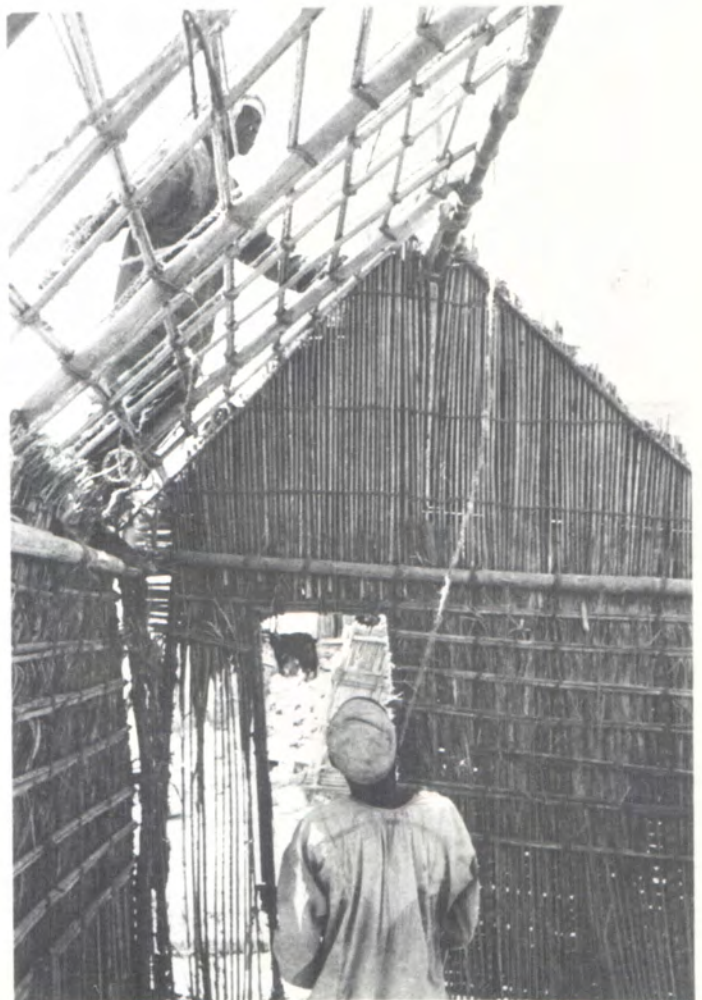
Fig. 835 The roof is post tensioned and tied when in place
