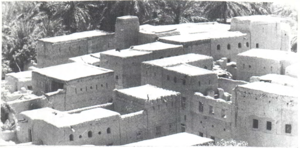
Construction of the traditional Flat Roof becomes a problem when timber is expensive or unavailable.
