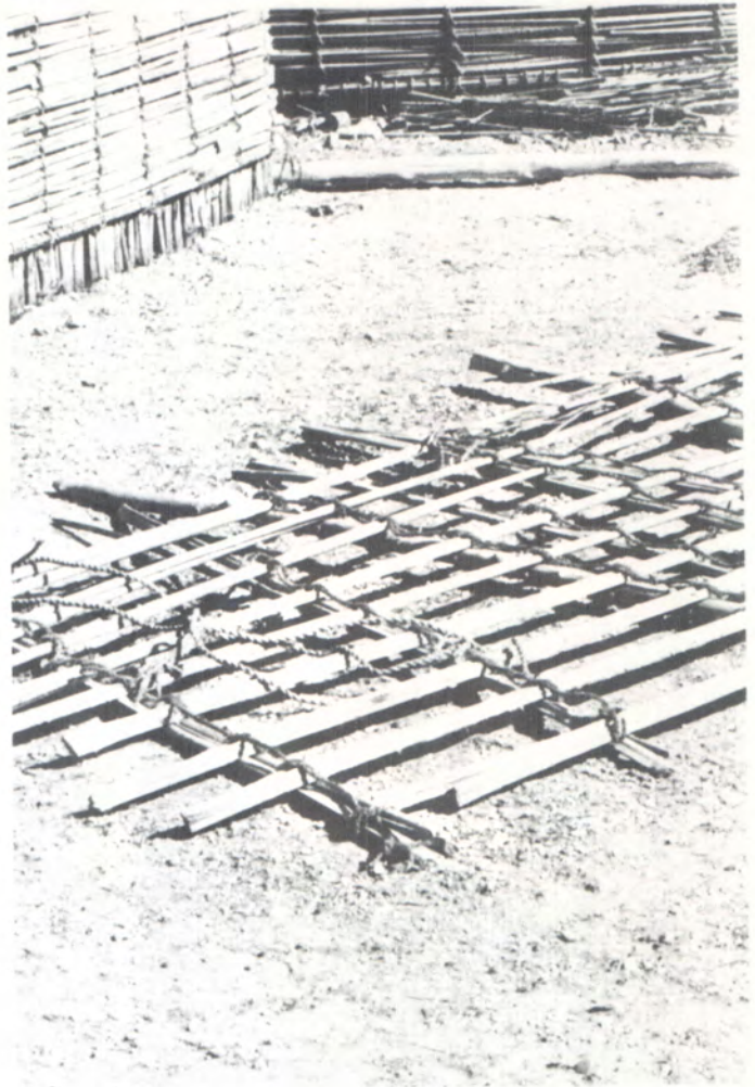
Fig. 834 The basic roof structure is pre assembled on the ground
